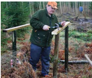
Kojans underrede tar form.
